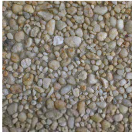
Silica Aggregate Concrete Mix: Exposed
